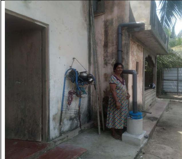
Kanagalingam Ramesh, well and well recharge system
