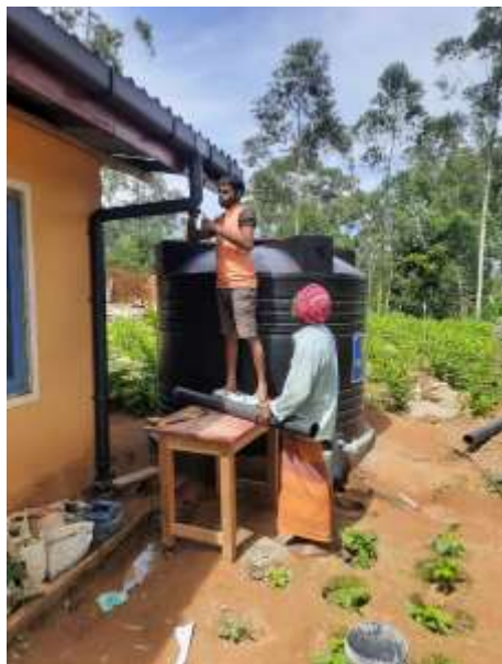
RWH under construction by the trained mason ( Son in Law)
