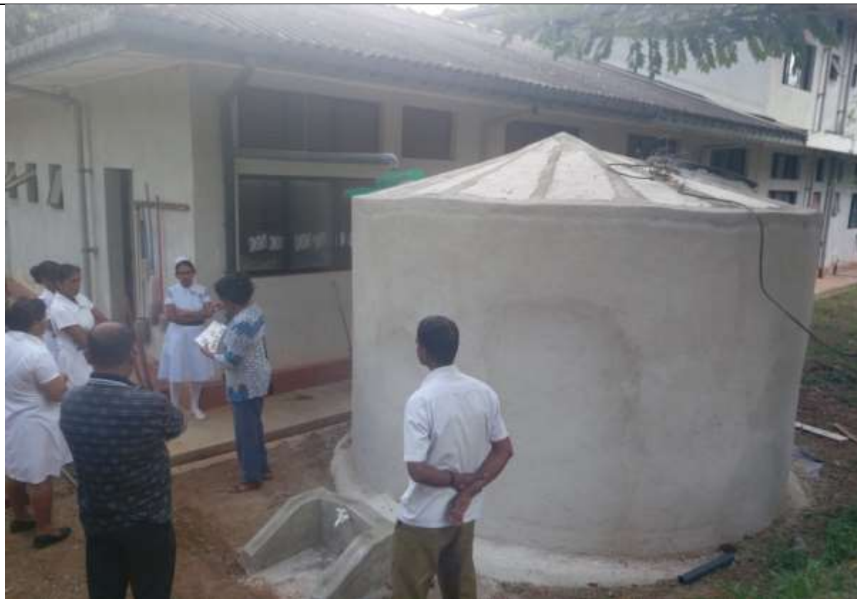
16,000 L Wire Mesh RWH systems with first flushes, filter and tap stand
