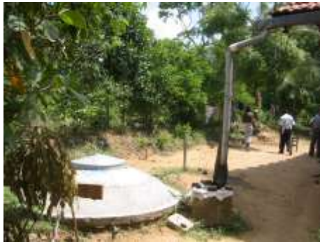
Figure 6: Brick under ground tank: 5m 3 capacity Constructed with brick and cement
