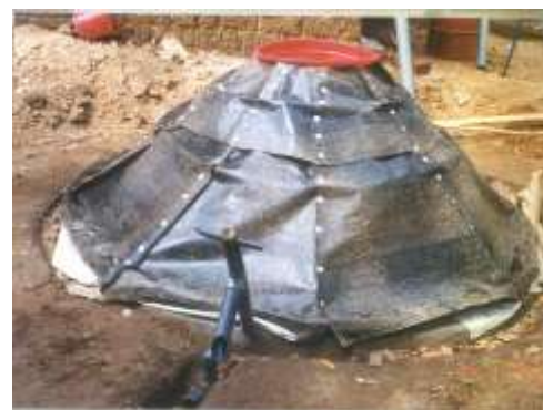
Figure 9: Thatched under ground tank: below ground is cement and chicken mesh and above ground cover is of tar sheets
