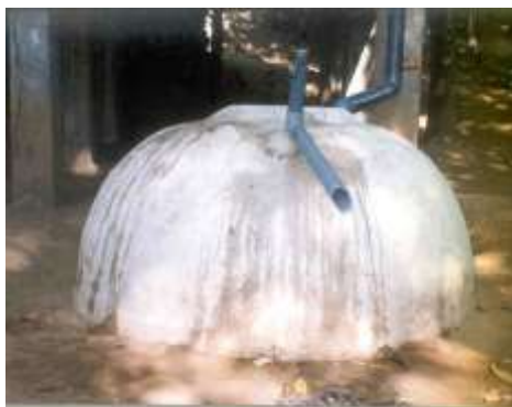
Figure 8: Ferro-cement partial under ground tank: Constructed with Cement and chicken mesh
