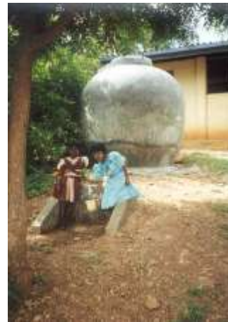
Figure 7: Ferro-cement Above ground tank Constructed with chicken wire and mesh
