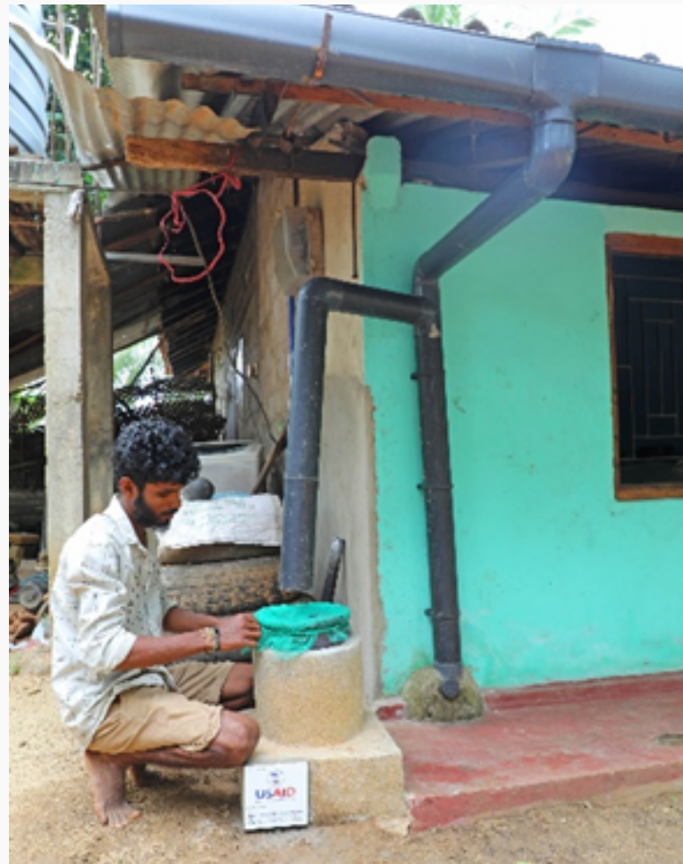
Well Recharge System at S. Selvarasa's home
