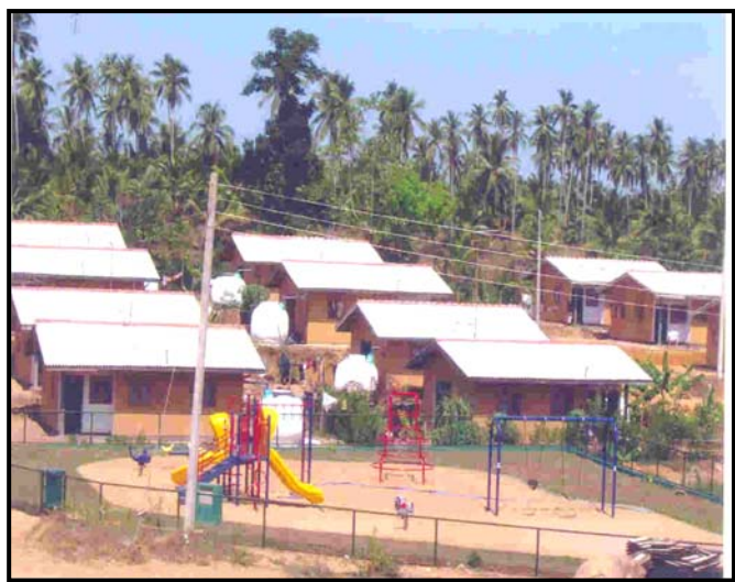
Rain water harvesting tanks in Rathgama – Nisalasewana (Tsunami housing scheme)
