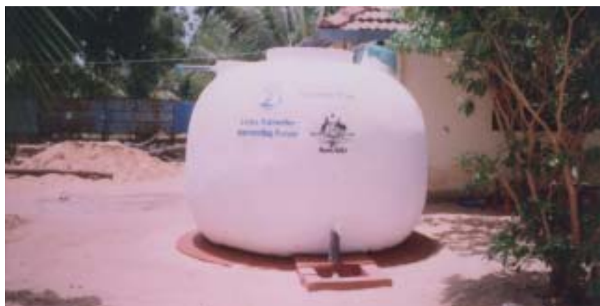
▲ Demonstration Rain water Harvesting Tank at NGO Consortium, Mullativu
